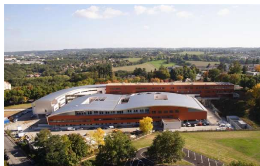
Nantes St-Jacques Hospital, France
