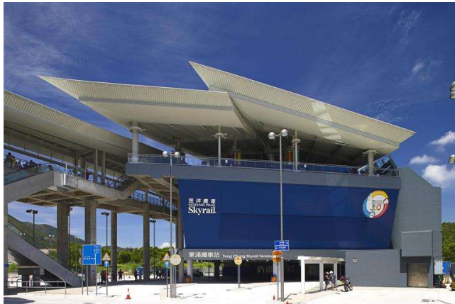
Tung Chung Cable Car, Hong Kong
