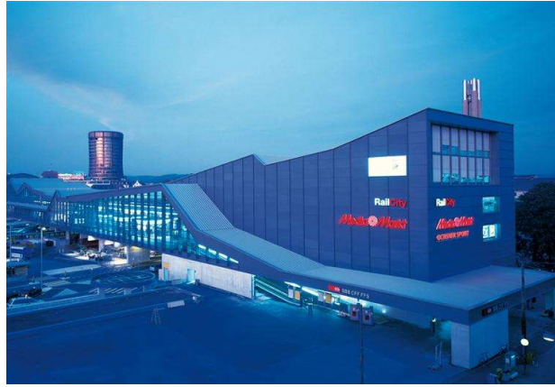
Passarelle SBB train Station, Switzerland
