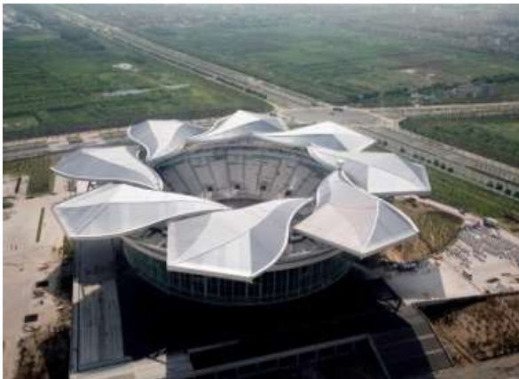
Qizhong Tennis Centre, Taiwan
