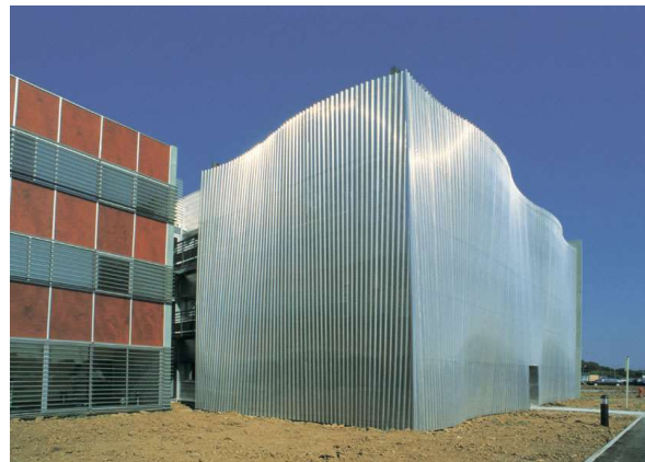
Dell Computer Centre HQ, Germany
