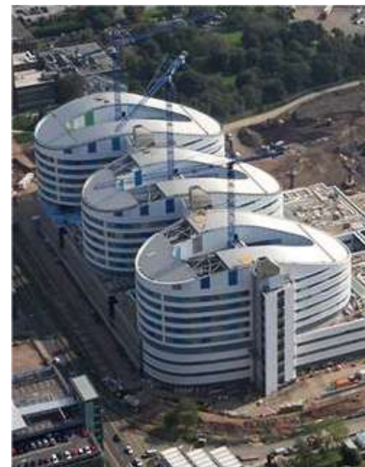
New Birmingham Hospital, UK
