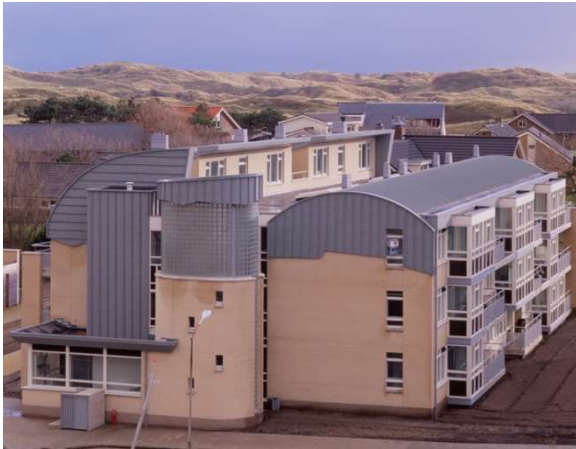
Woningen Torenduin Egmond aan Zee Residential housing, Netherlands
