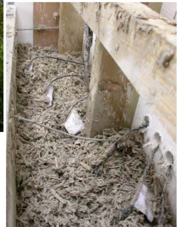
Figure 3: Sensors embedded in the hemp-lime wall during construction
